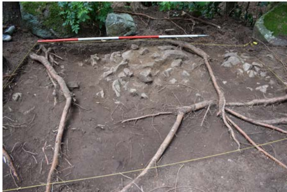
Plate 25: Stone demolition material (117) over wall (125); facing west, note the root tracks which have damaged the structures and moved stones
