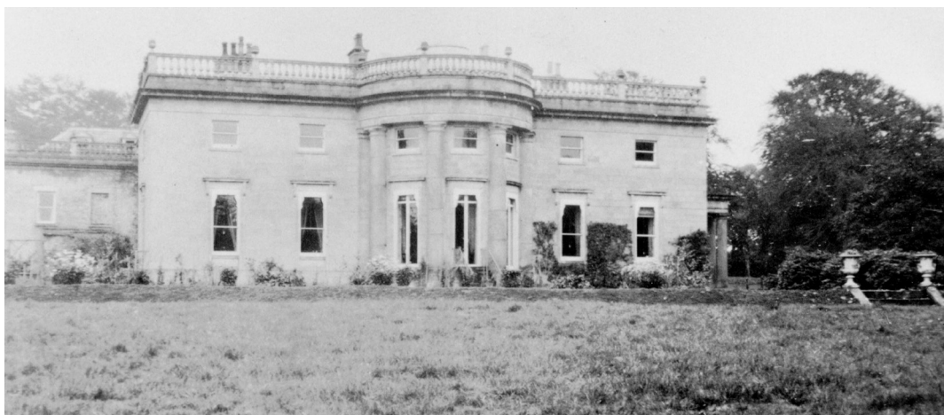
Plate 51: Mid-twentieth century photo of west façade of Aden House (Courtesy of Aberdeenshire Council)
