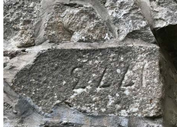
Plate 44: 1773 incised date stone reused upside down as the springer for an arch; facing west
