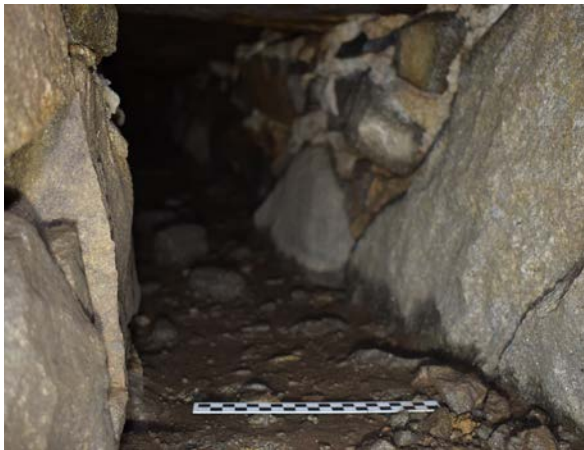
Plate 54: Trench 11 drain (1109) east wall mortared into the mansion's west wall foundation
