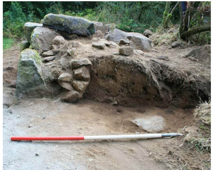
Plate 68: South façade of wall (539) showing soil infill behind steps and no evidence of steps on south side of wall; facing north
