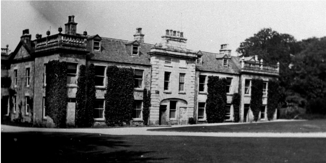
Plate 60: Cart door (centre) showing infilling with stone and brick wall (1703); facing NE (@ Aberdeenshire Council)
