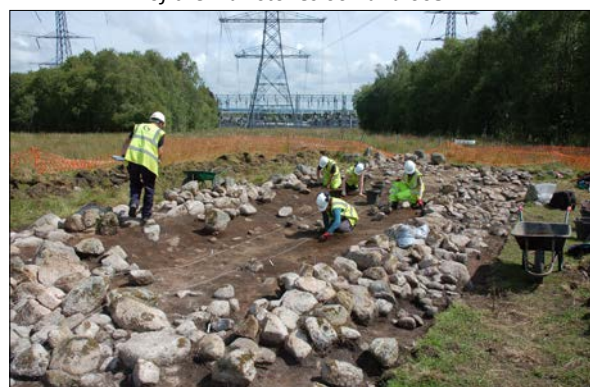
Plate 2: Working shot of during excavation of the walls and interior of the building.
