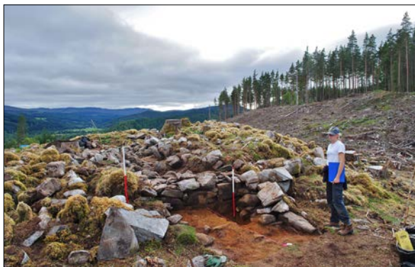
Figure 9: Looking south-west over the outer wall (201) and Trench 2.
