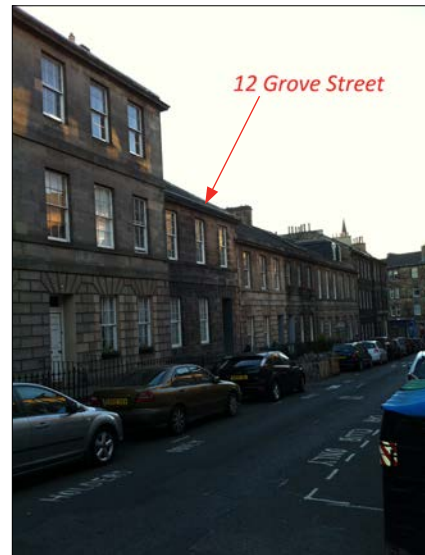
Plate 1: Terraced housing at Grove Street.
