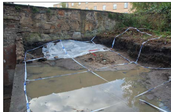
Plate 2: Pre-excavation of site.
