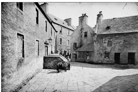
Plate 4: Commercial Street, Lerwick: the dark bituminous stain is evident in the gable end below the chimney (© Shetland Museum and Archives).
